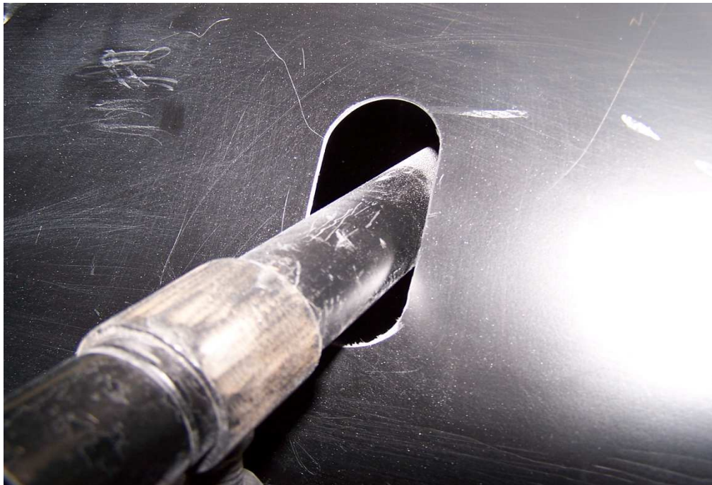
Marking out for cutting hole through bulkhead
